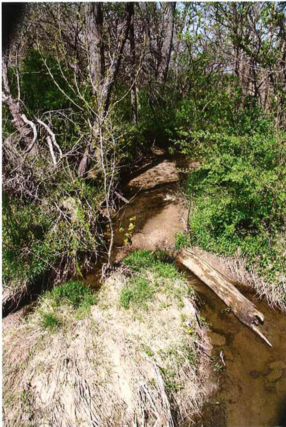
Site US51-68. Unnamed tributary (e) of Vandalia Lake, at the Illinois Route 185 box culvert, 3.7 mi (6.0 km) SW Vera (town). Looking upstream / north. Photo by M.J. Wetzel, 14 April 2011. [ a downstream photo follows... ]
