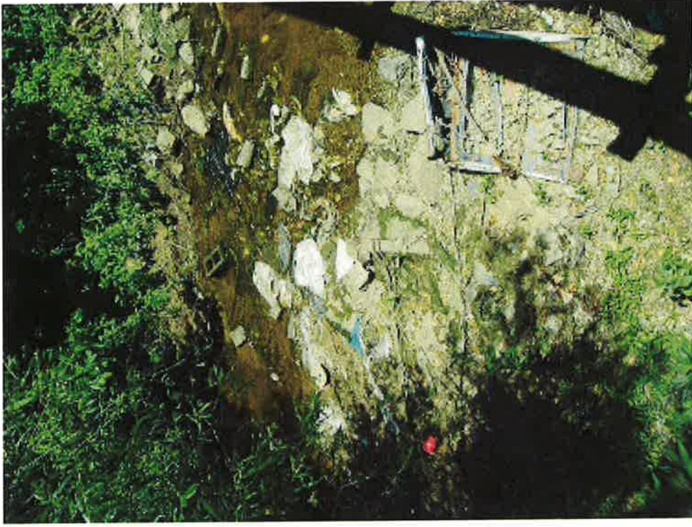
Figure 13. USS1-53, Prairie Creek, at Barton Road bridge, 1.4 mi SW Sandowal – 29 June 2009. Looking downstream (W) of bridge, showing accumulation of junk, garbage, and fish carcasses that had been dumped here.
