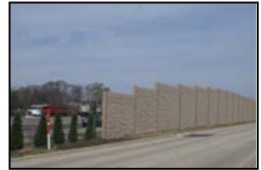
Noise Wall (photo courtesy of IDOT)
